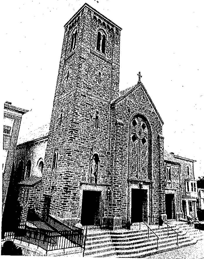
Immaculate Conception Church Exterior with Ramp installed in 1990.
